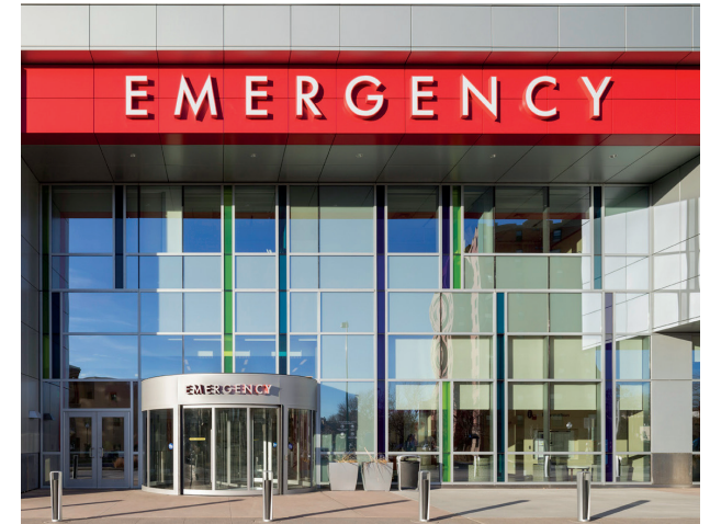
HSS adjusted its security plan to accommodate design changes such as adding a metal detector to the hospital's new ED.
